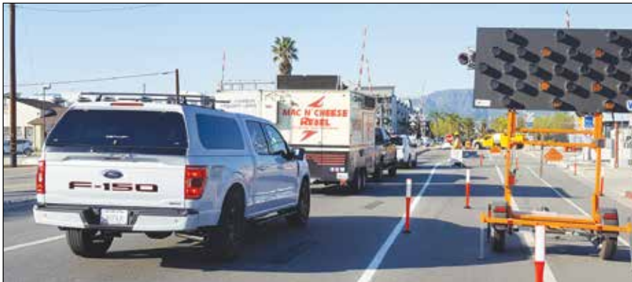
TRAFFIC ON GAREY -- A worker, pictured four cars up at the tracks, holds up a "stop" sign while construction workers move equipment around at rear to do a little digging in the street as they work on relocating underground utilities in preparation for getting the tracks ready at the Garey Avenue crossing for the Gold Line light rail project extension. Also visible is the white line "restriping" that narrows Garey down to one lane in each direction in a project that will continue until the end of the year.
