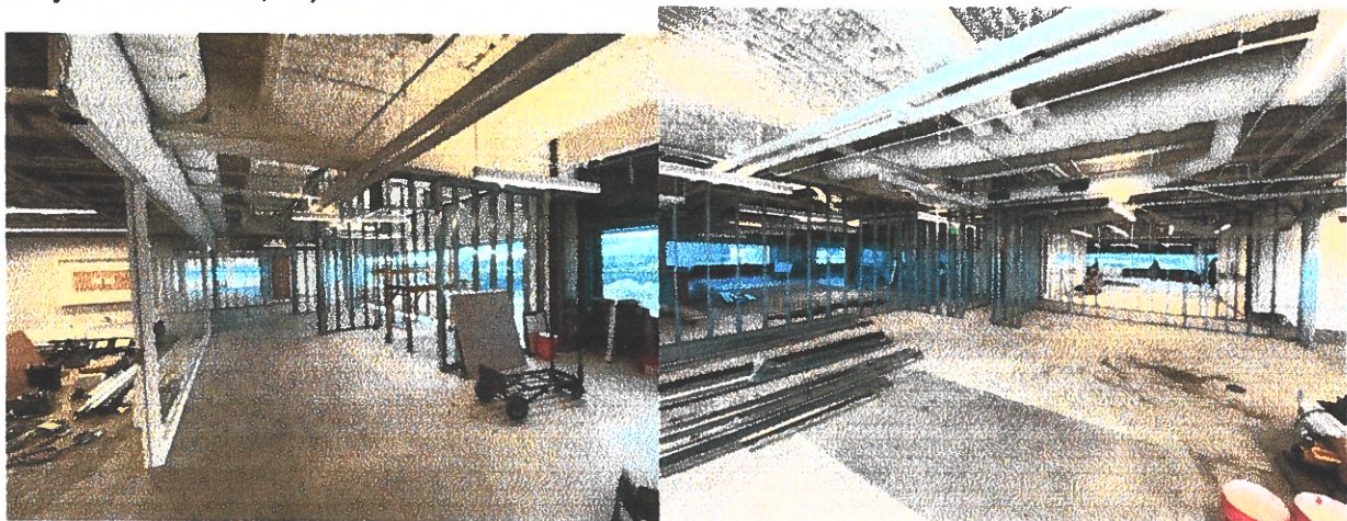
2101 E El Segundo Blvd 5 th Floor – Framing Project Amount - $60,000
